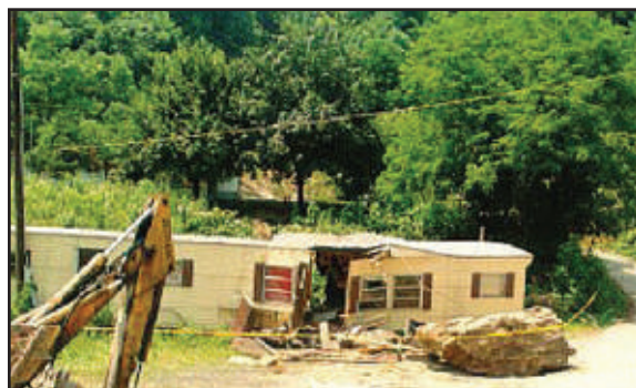
In areas of steep slopes, a rock set in motion by the explosive energy may roll hundreds of feet. This rock rolled through a trailer downslope from a mine.
