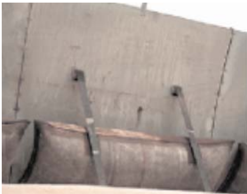
Photo 5.6: Flashboard controlled by inflatable rubber bladder
