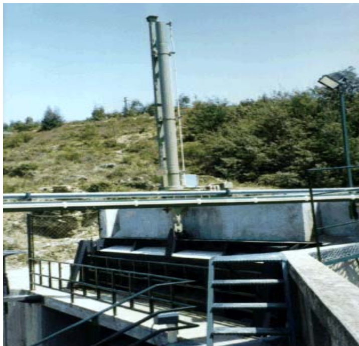
Photo 5.12: Hydraulic Cylinder
