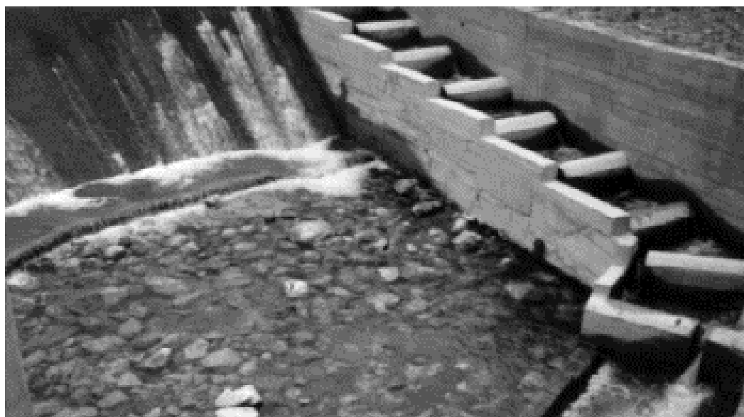
Photo 7.14: Fishpass with vertical slots
