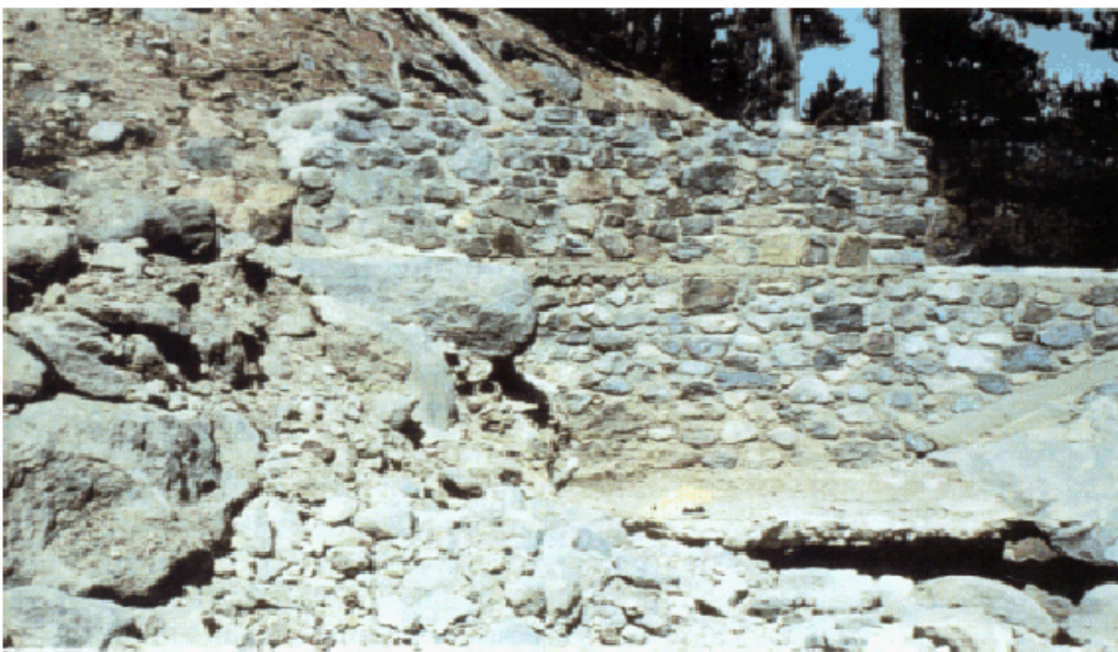
Photo 4-11 Weir undermined by seepage
