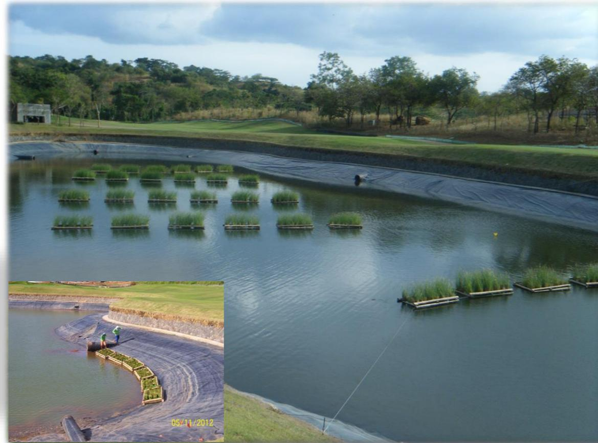
**On manmade ponds and lagoon for effluent control**
