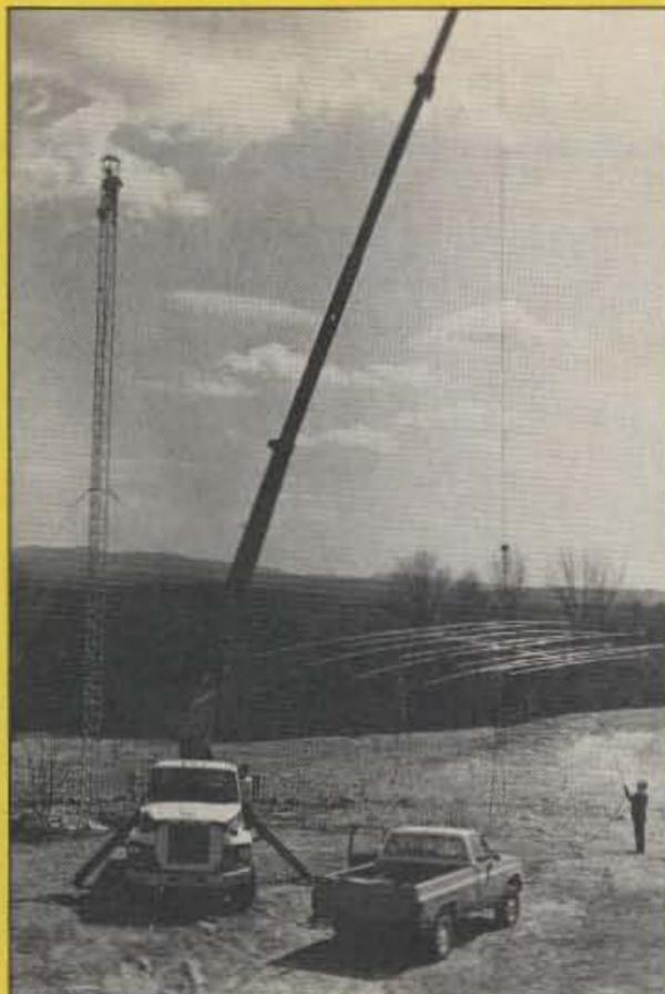
*What new station would be complete without a new tower and antenna system. W2NSD's latest toy is a Sommer multiband HF beam sixty feet up.*
