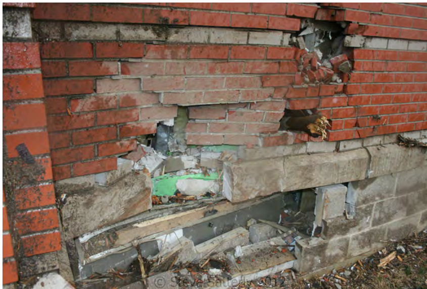
This is a major impact scar from a large object. It also shows a tree branch that pierced the side of the school, and a hole in the upper right caused by a debris missile.
