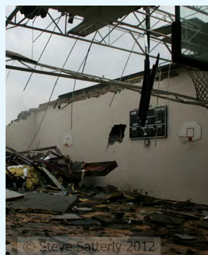
This picture of the Henryville Elementary School gym shows a missing roof, the collapsed wall, and the impact hole next to the scoreboard.
